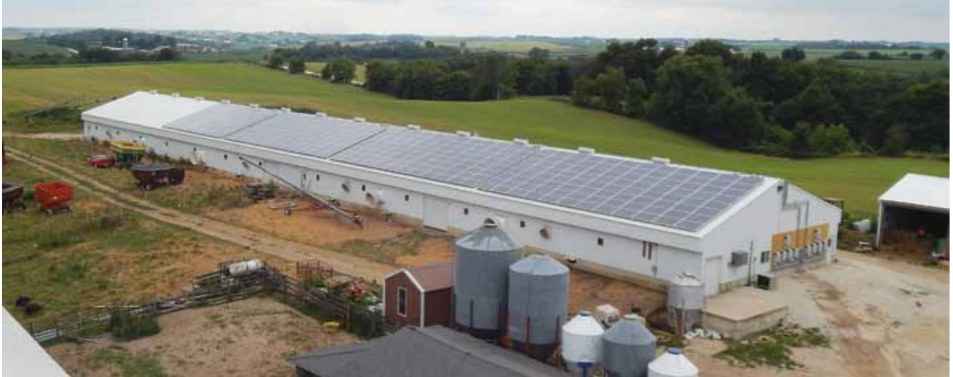
This 360-panel solar array in northeast Iowa generates enough power to reduce the poultry farm's utility bills by 90%.
